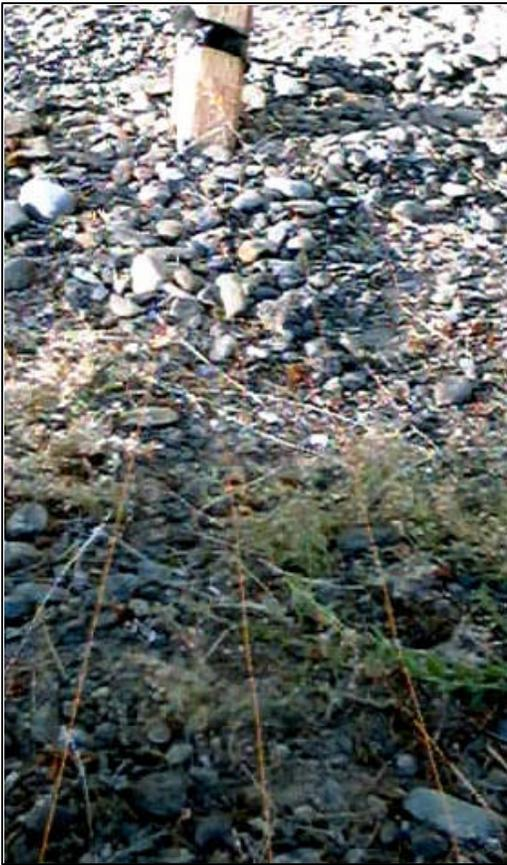
10 wire radials measuring between 40 to 80 feet in length were buried 1 inch under the gravel and then attached/soldered to a 3 inch x 2 inch piece of copper plated circuit board. The board was then connected to the braid side of the coax which was in turn connected to a ground rod, sunk 6 feet in to the earth next to the feed line.
